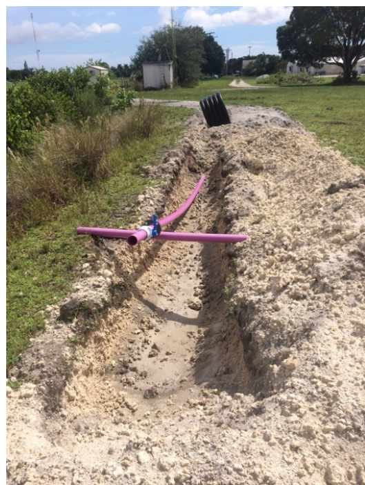
Picture 1. Four inches main line purple pipe brought to FLREC from Town of Davie Water Treatment and Water Reclamation Facility that is going to feed the research plots
